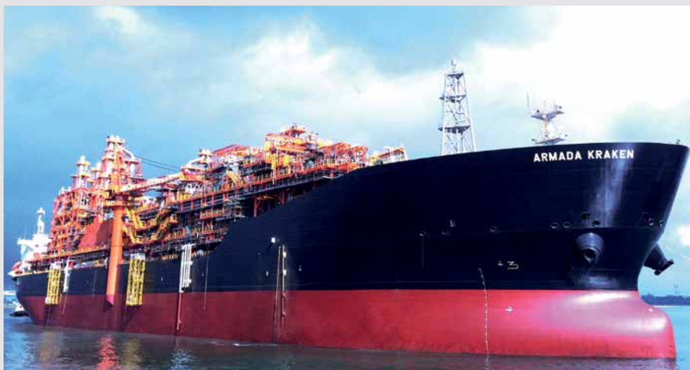
Armada Kraken is a complex harsh environment FPSO which meets the stringent requirements for the UK North Sea
